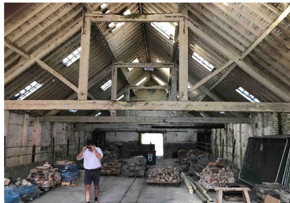
Internal view of central barn range (plots 4)
