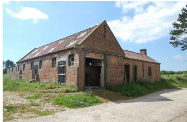
Stables from north east
