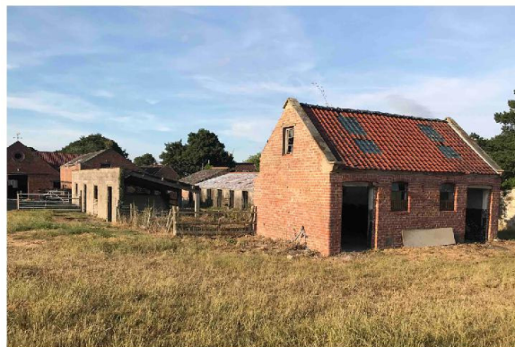
South west side of Home farm outbuildings (plot 1)
