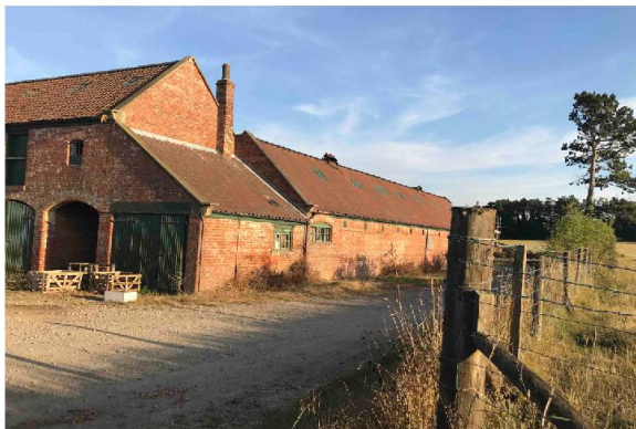
Barns north west corner (plots 4)
