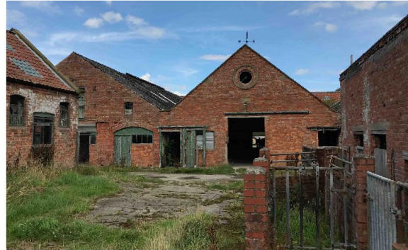
South view of central barn
