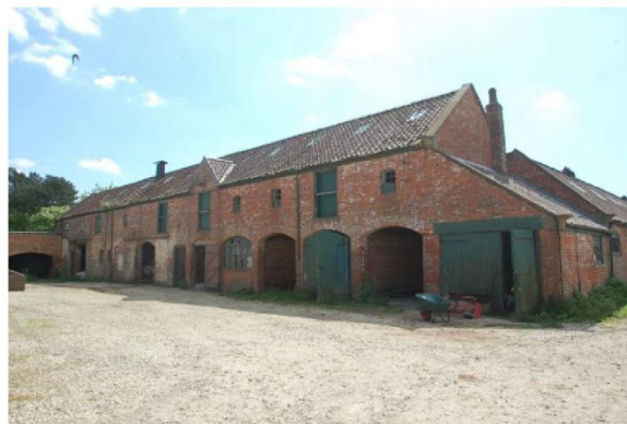
The barns north elevation (plots 4)
